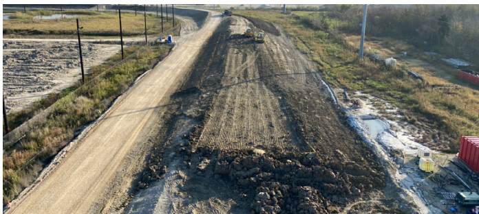
A section of raised levees under construction in Port Arthur
